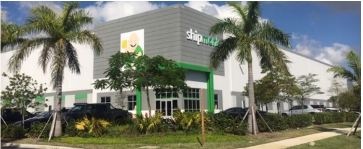
Shipmonk Completed Project - 201 NW 22 Avenue
