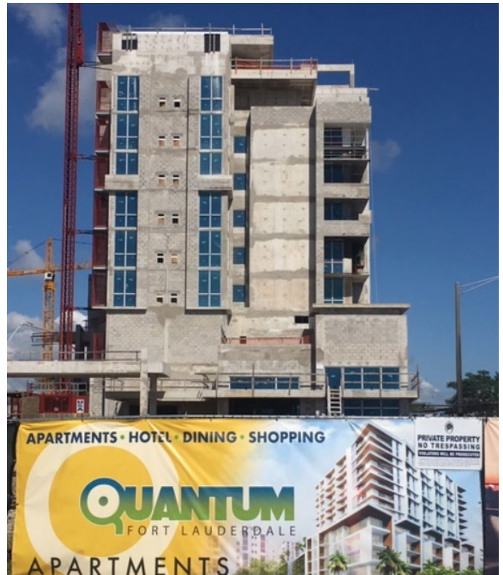
Construction of Quantum Fort Lauderdale
