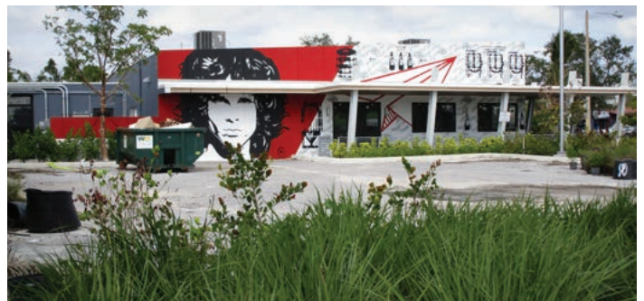
914 NE 4 Avenue restaurant/bar/brewery
